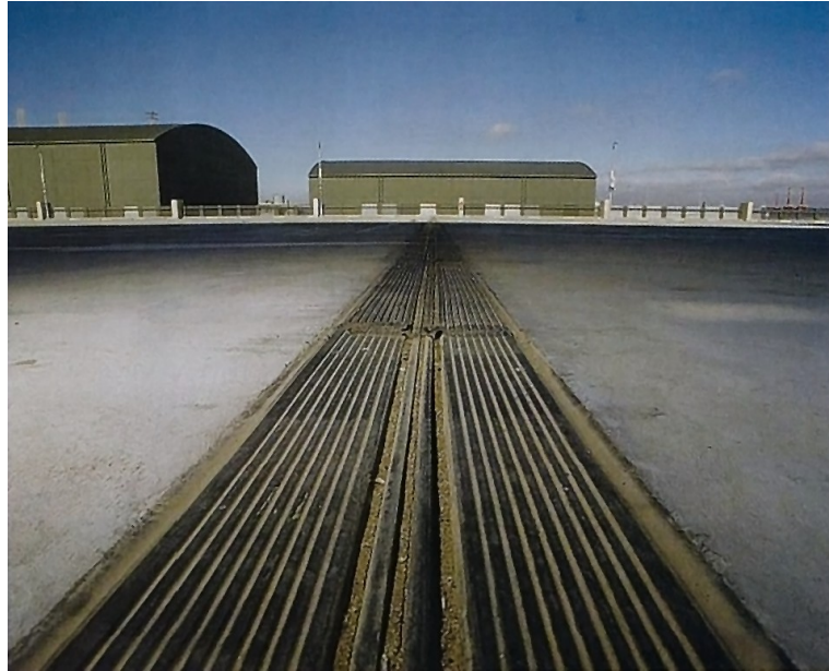
This high performance expansion joint was recently installed on a car park at Waterfront City development in Melbourne's Docklands.
